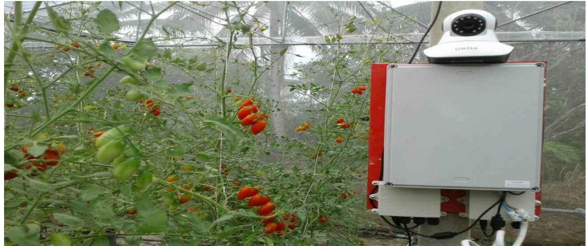
Control system testing
